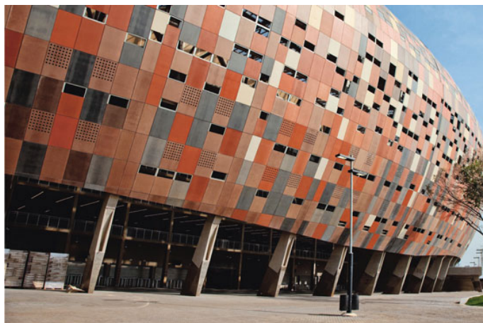
Photo: Soccer City Stadium, Johannesburg; made of glass-fiber-reinforced concrete colored with Bayferrox pigments. Source: www.bayferrox.com
